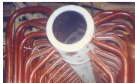
Header ligament cracking
